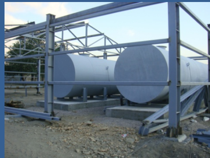
Adsorption, cyanide, water and pregnant solution tanks
