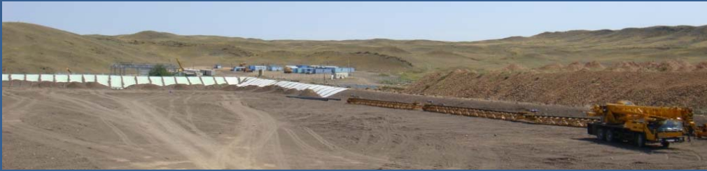
Conveyors ready for installation on heap leach pad
