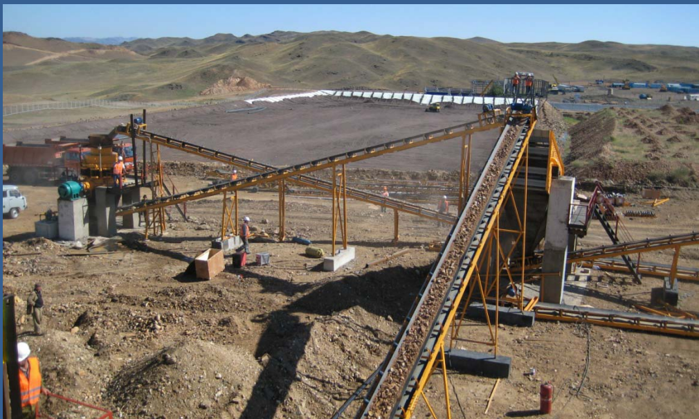
Successful testing of crushers and conveyors
