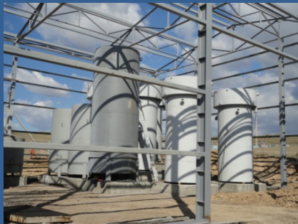
Adsorption, cyanide, water and pregnant solution tanks
