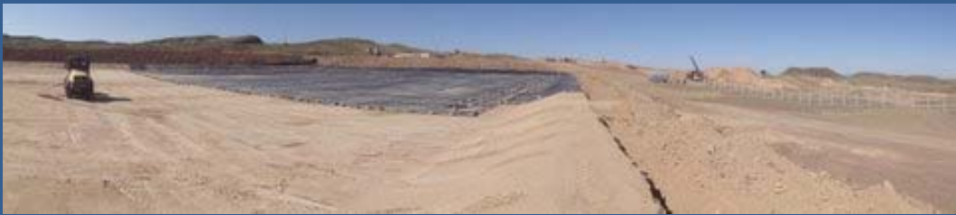
Leach pad lining partially laid
