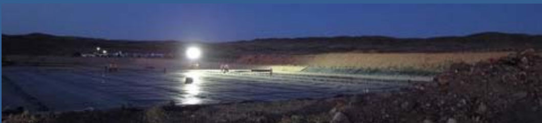
Laying leach pad lining
